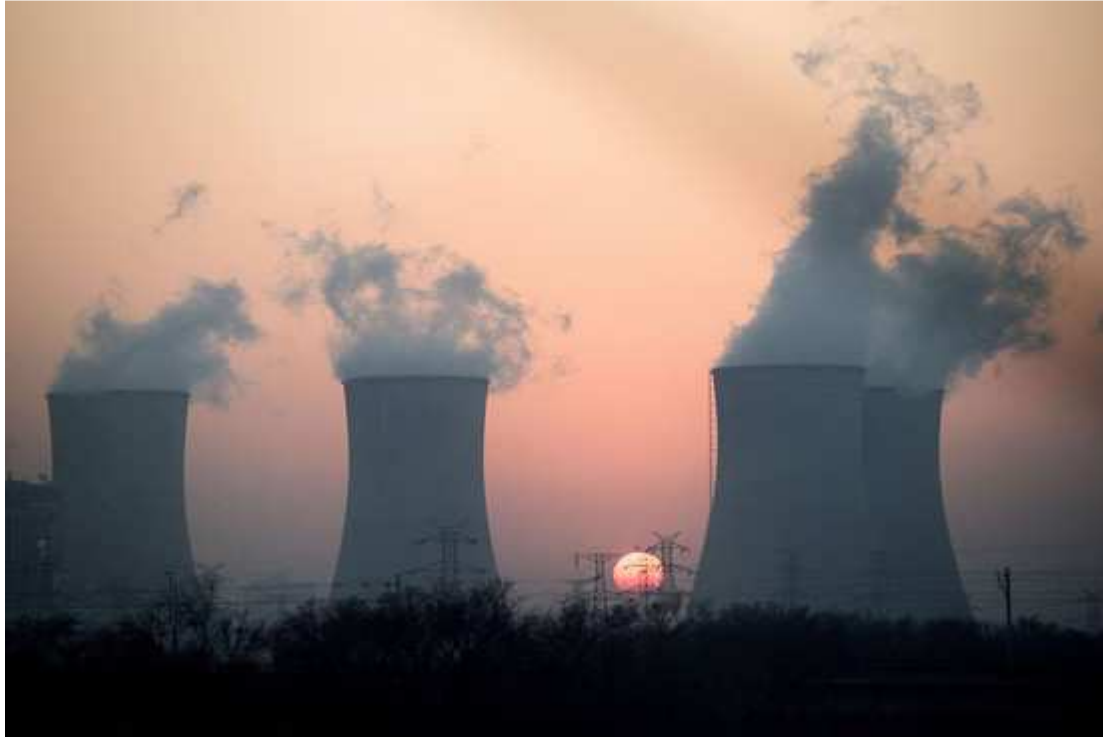
A power plant near Hengshui in China's Hebei province.- Agence France-Presse/Getty Images
